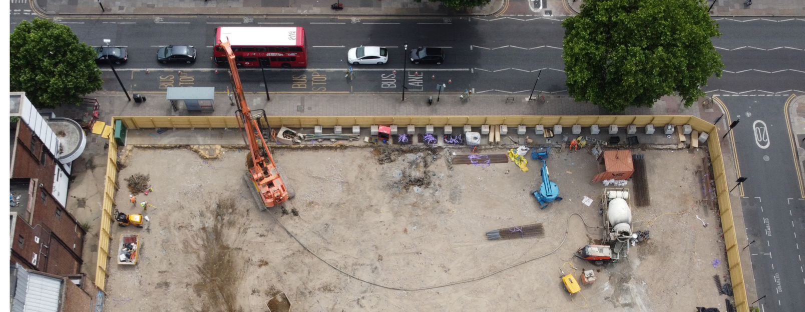
Image (right) : Site Preparations at the Hartley Centre in 2022
